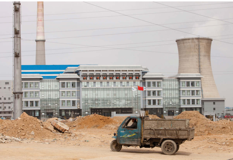
Coal-fired power station in China
